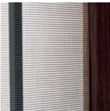
033 Windows and French windows have sliding wooden panels with fine nylon screens to provide protection from mosquitoes and insects.
