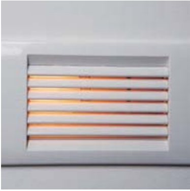
041 Footlights provided at convenient locations in rooms and passages show you the way at night.
