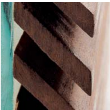
035 Bathroom doors have wooden louvres with glass panels that let in light without compromising privacy.
