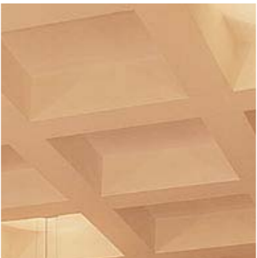
028 The use of coffer slabs eliminate the need for conventional beams and result in dramatically enlarged spaces.
