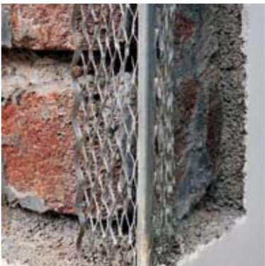
031 A GI mesh is embedded along corners of walls while plastering. This prevents chipping of edges and goes a long way in keeping the walls in great shape.
