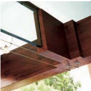
025 The glass deck on the upper level is supported on extra strong PVB laminated glass structural beams. The floor panels themselves can take a load of upto 1.5 tonnes.
