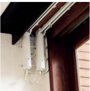
036 Draw curtains by simply pressing a button. Remote activated curtain-controls add a whole new level of convenience.
