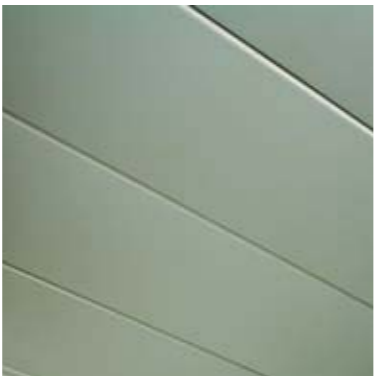
027 The false ceiling enhances the visual appeal of bathrooms and keeps service ducts concealed.
