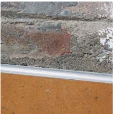
030 An aluminium U-channel is provided between the floor-skirting and the plastering of the wall for better finish. It also conceals cracks that may develop due to expansion.
