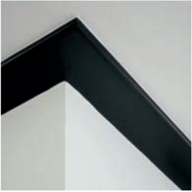
046 Wooden cornices that run along the ceiling conceal fire-fighting sprinklers even as they provide better finish to the rooms.
