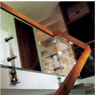
026 Cantilevered steps and tempered glass create a sense of lightness and transparency about the stairway. The handrails are crafted out of high grade teak wood.
